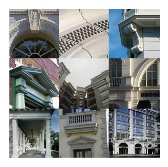
Glass fiber Reinforced Concrete, also known as GRC, is made of alkali-resistant glass fiber as a reinforcing material. Sulphate-aluminate low-alkalinity cement is used as a cement material and is mixed with suitable aggregate to form a substrate. Lightweight, high-strength, high-tough, multifunctional new inorganic composite materials made by casting, extrusion, and slurry production.
